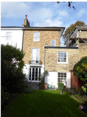
Rear elevation (North) and garden
